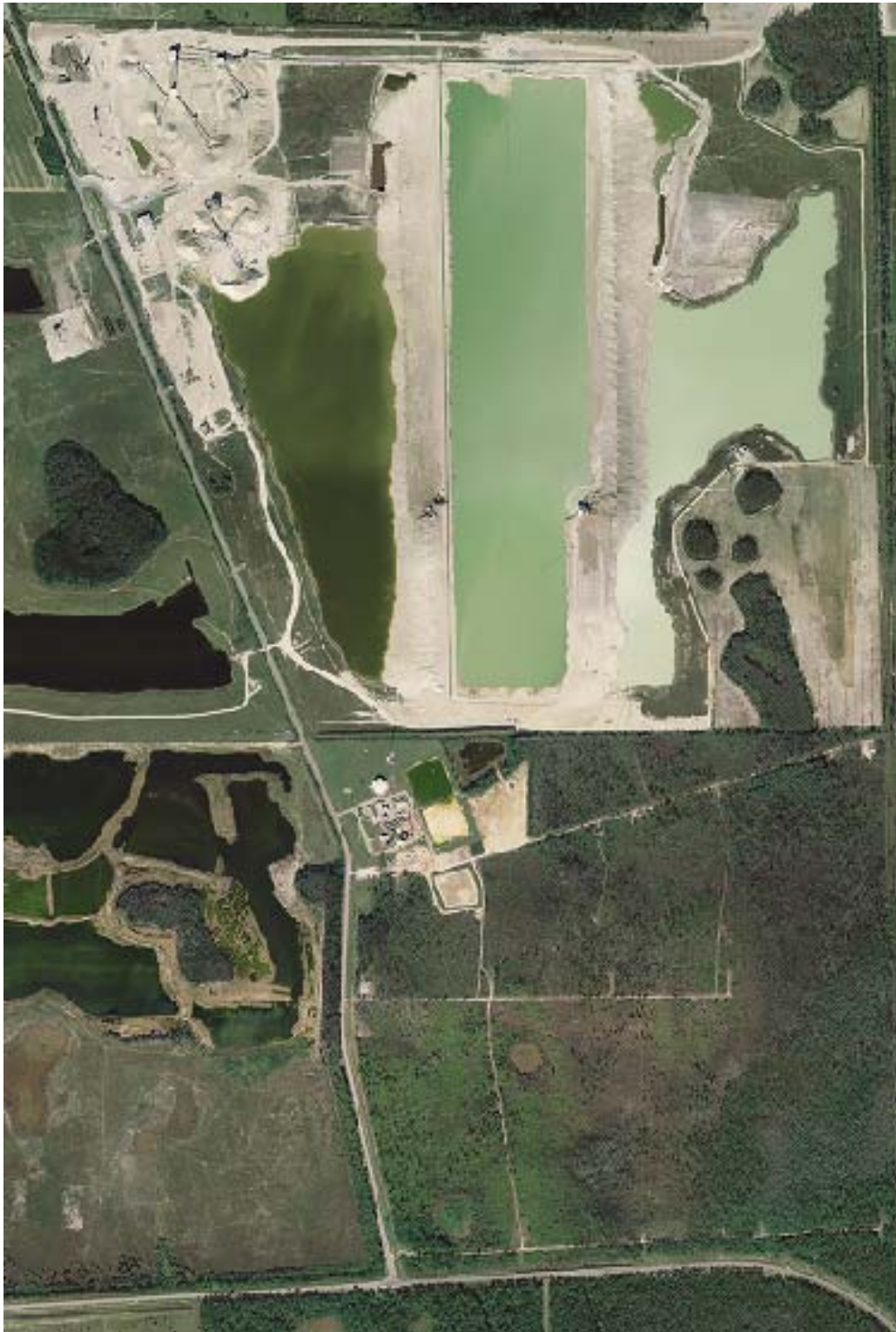
Figure 1 – University Lakes Mine and Corkscrew Water Treatment Plant & Wellfield
