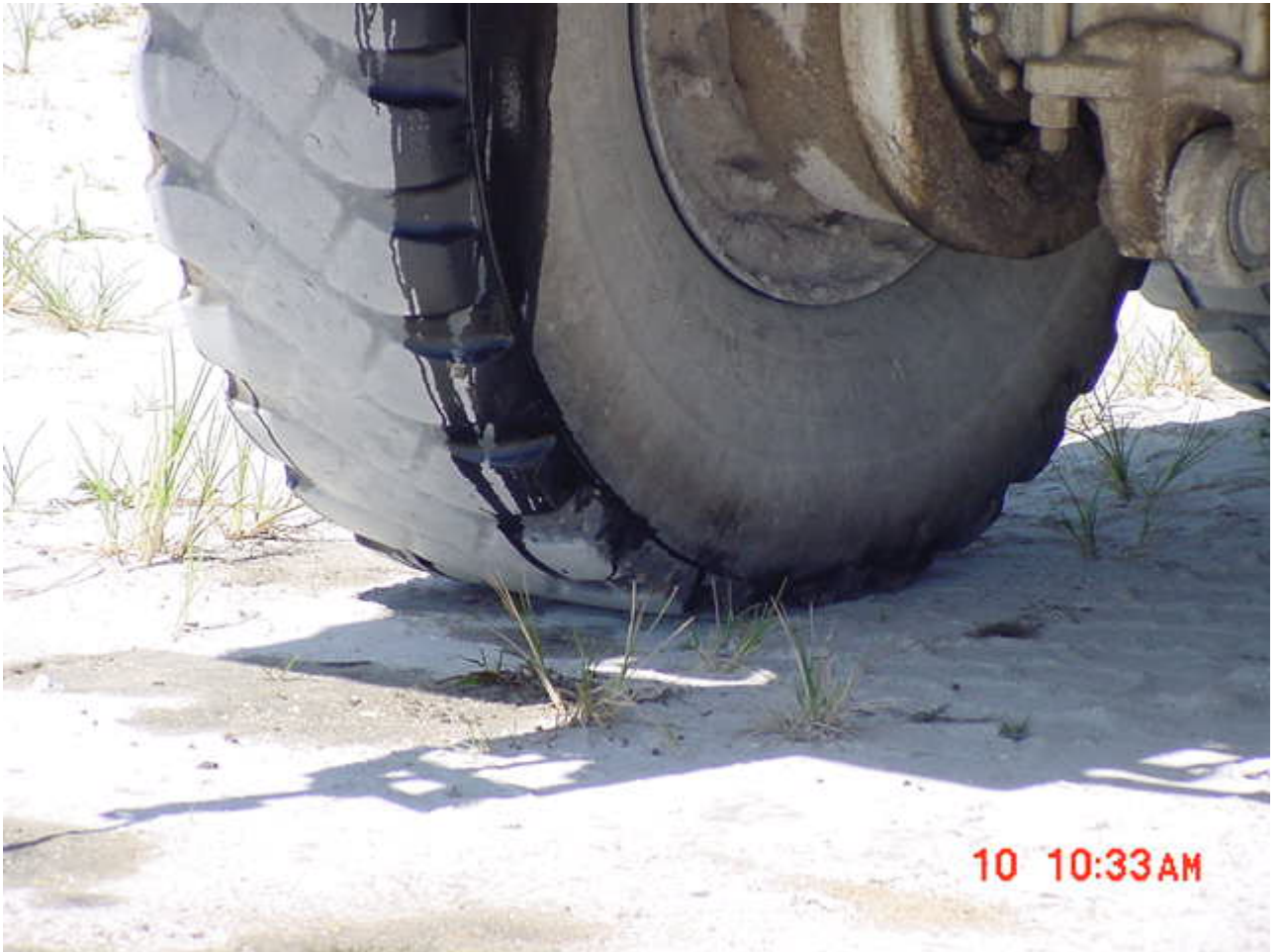
Evidence of one of the leak's from fueling vehicle running down the left rear tire onto the soils.
