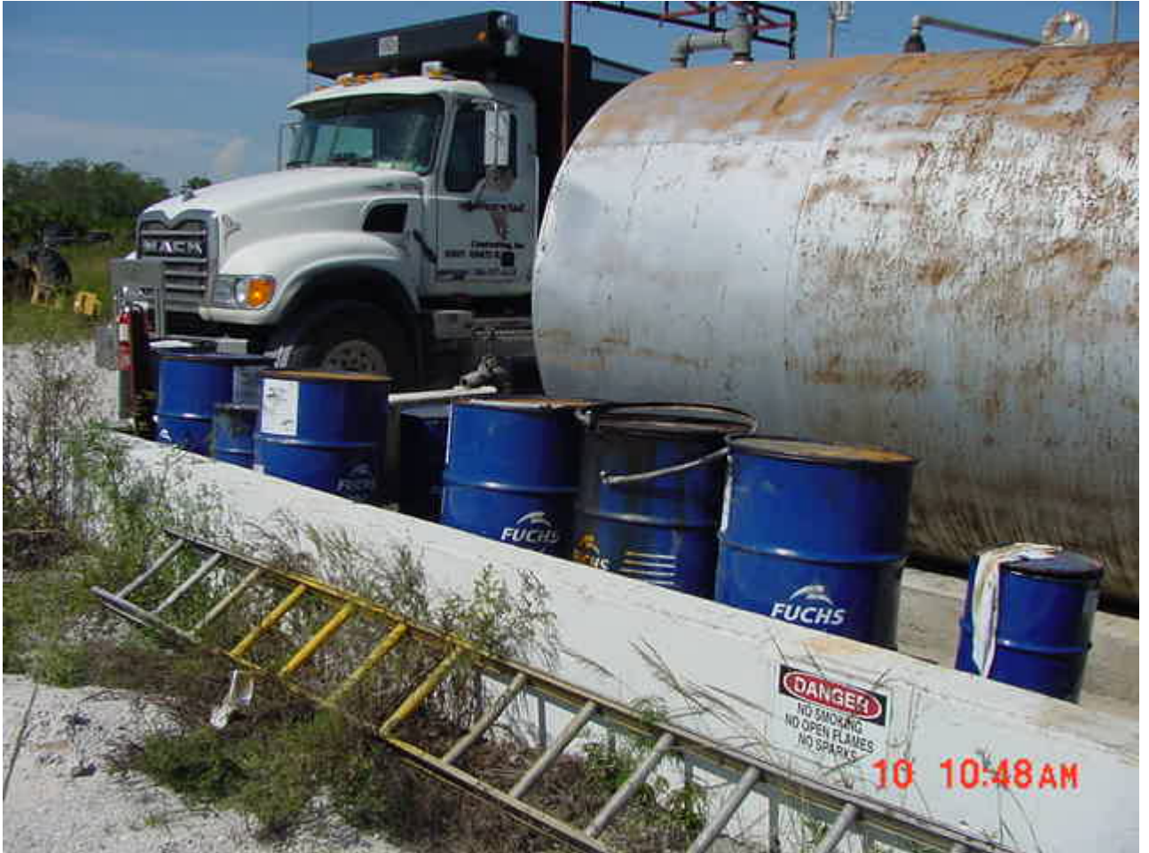
Under the ladder within the stressed vegetation is evidence of petroleum discharge along east wall of containment system.
