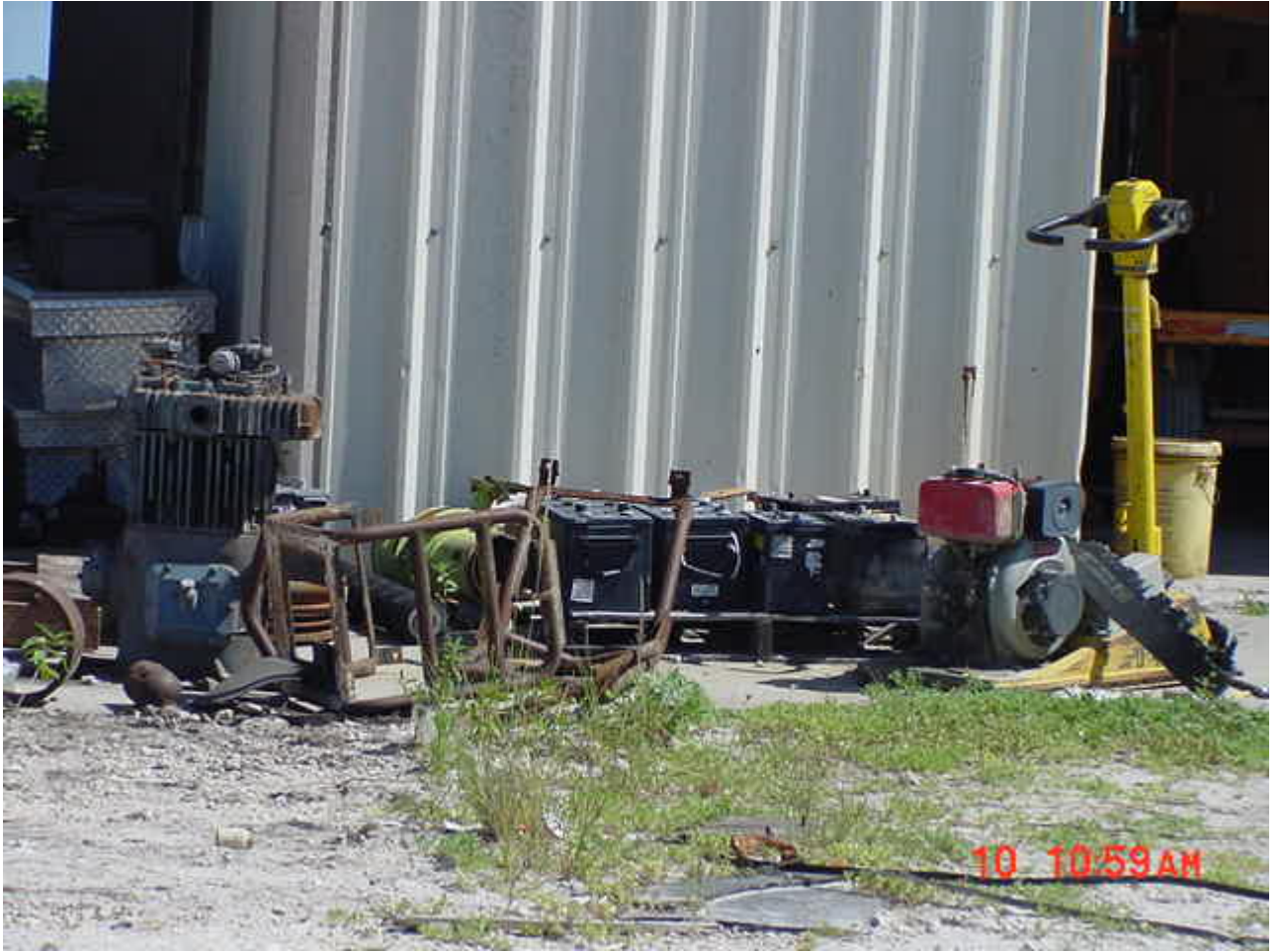
Lead acid equipment batteries stored outside of building within the drip edge of the roof and not within containment to protect from contaminated rainwater runoff. Stained soils in various places along perimeter of building.
